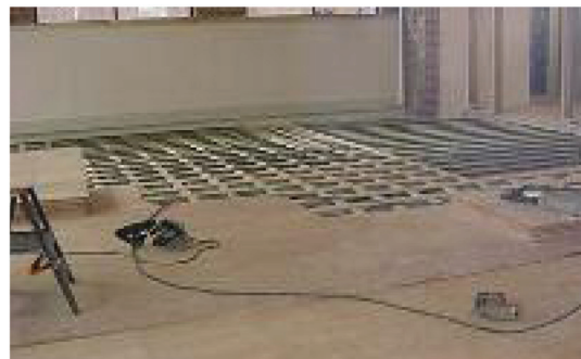
Installation of Harlequin WoodSpring at the Boston Ballet School
