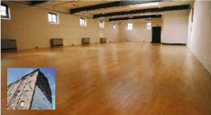
New Activity Floor with maple surface installed at New Cut Arts Centre, Halesworth, Suffolk.
