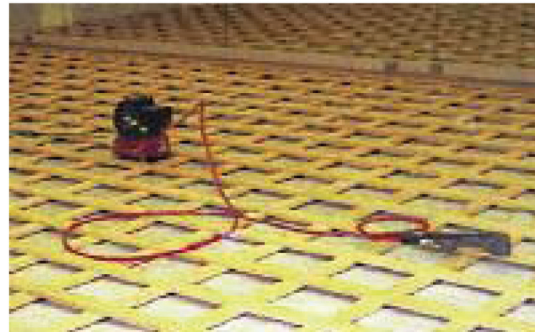
Completion of first and second layers of basketweave structure
