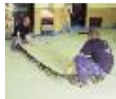
Top semi-flexible panel layer with joints staggered
