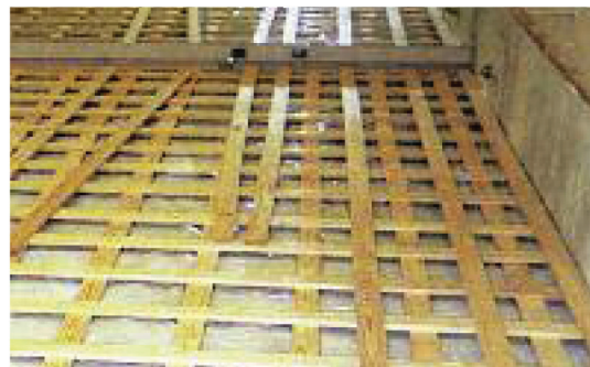
Installation of third layer in progress
