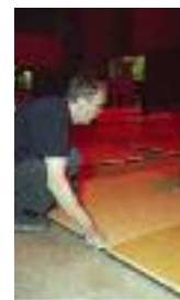
Installing the panels
